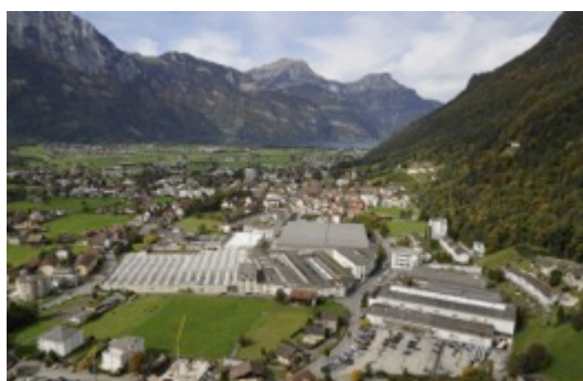
Dätwyler Cabling Solutions AG Altdorf
